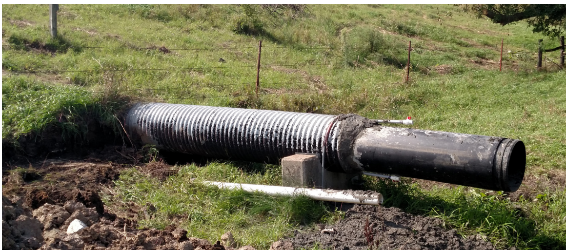
Johnson 46 structure renovated with Slip-Tite lining in summer 2019.
