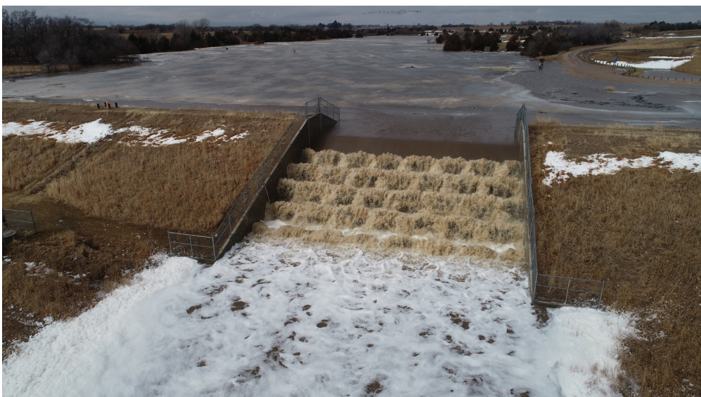
Flood waters controlled by NRD structures in York in March (left) and in Aurora in May (right).
