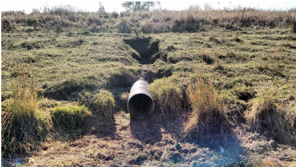
NRD staff repaired Dunker Dam near Ulysses in 2021 (left)
