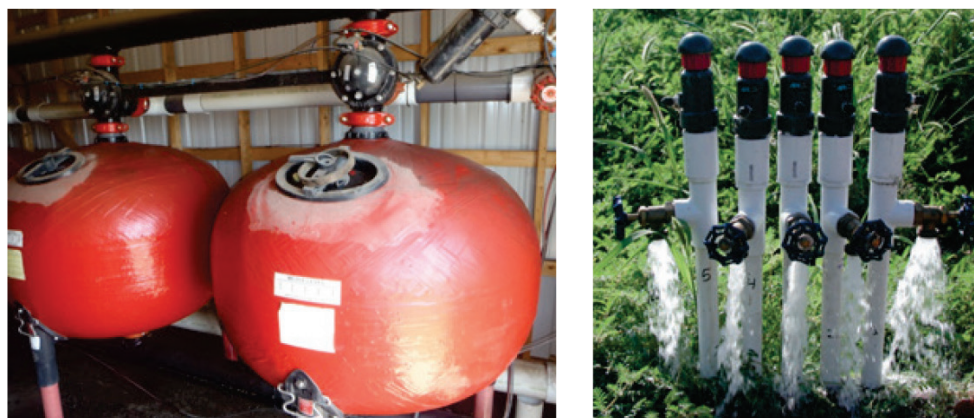
Figure M-4. Typical filtration system (left) and flush valve installations for SDI systems (right).
