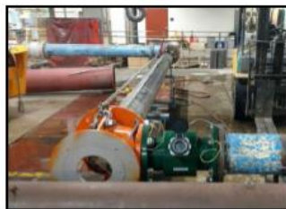
Zero Distance from Turbine Pump Discharge
