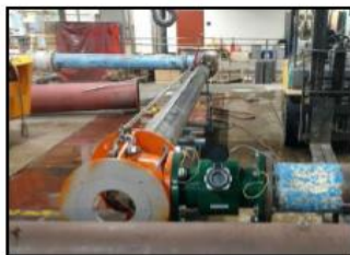
Zero Distance from Turbine Pump Discharge
