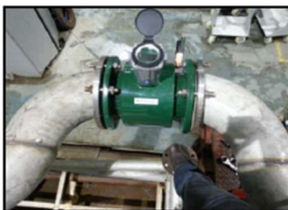
Zero Distance from Pipe Elbow
