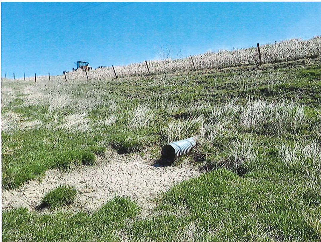
Bruner Road Dam – Pipe Outlet
