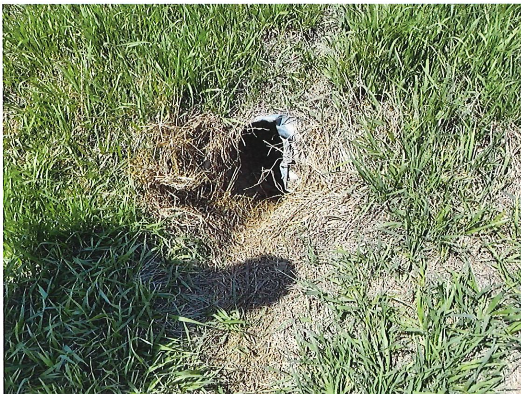
Bruner Road Dam – Damaged Pipe Inlet
