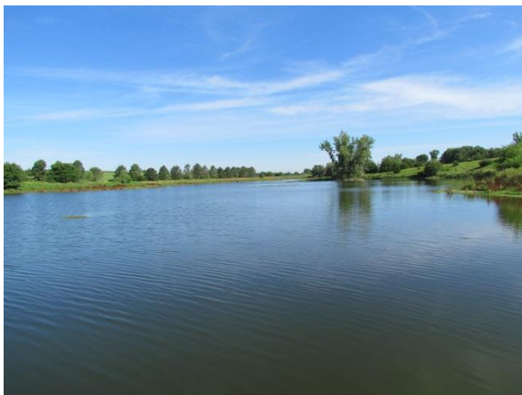
Lower End of Reservoir
