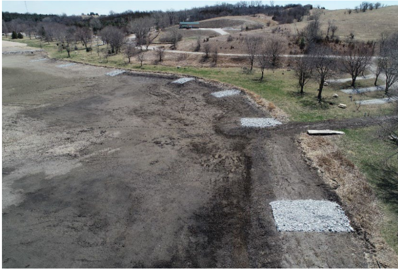
Figure 8. Gravel Spawning Bed. A combination of small riprap (Class A) and crushed limestone are placed in lake footprint adjacent to shoreline to block aquatic vegetation and provide fish habitat (photo from Summit Lake during lake drawdown).
