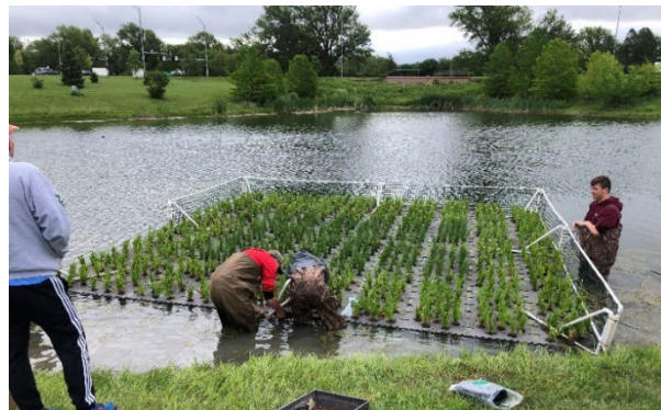
Figure 4. UNL Students assembling a floating treatment wetland at Cooper YMCA in Lincoln NE
